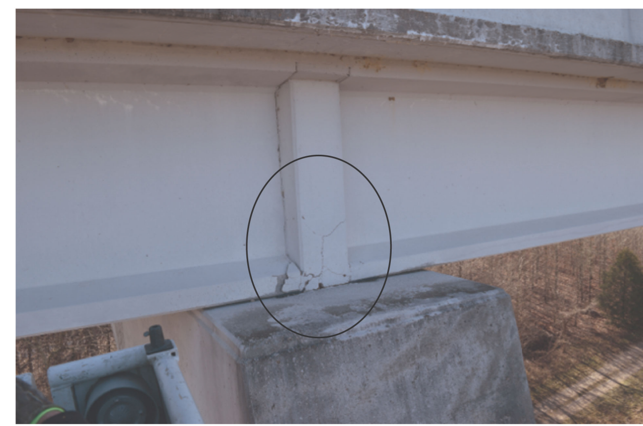
CLOSURE CRACKS - AT PIER 10, BEAM A (OTHER LOCATIONS SIMILAR)
