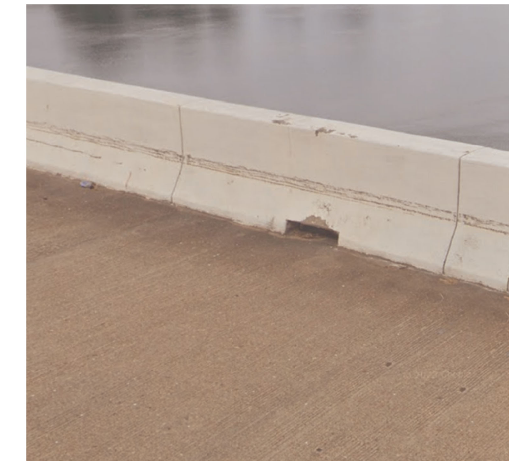
BRIDGE DECK DRAINS
