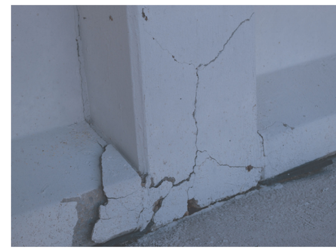
CLOSURE CRACKS - AT PIER 10, BEAM A (OTHER LOCATIONS SIMILAR)
