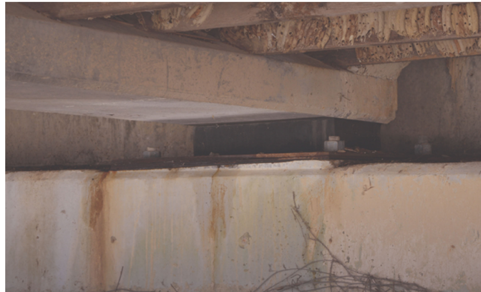
ABUTMENT 1 BEARINGS (TYPICAL BEARING SHOWN, OTHERS SIMILAR)
