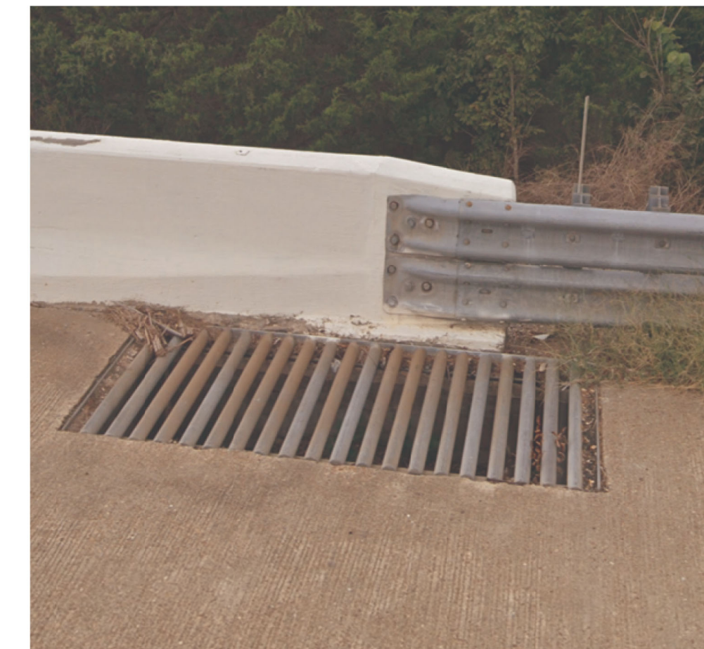
BRIDGE END DRAINS
