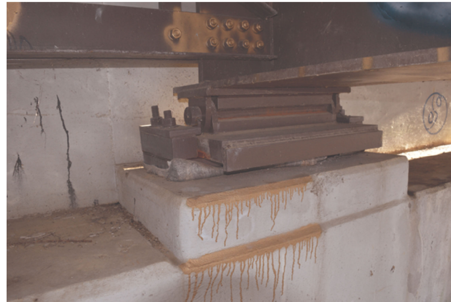
ABUTMENT 2 BEARINGS (TYPICAL BEARING SHOWN, OTHERS SIMILAR)
